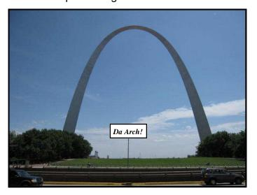
next to it and looks up. The sides are made of stainless steel panels and curve nicely to the top where they meet. I learned once on a cable history channel that when the builders went to hoist the last piece into position it would not fit. The fire department had to spray water on the high side and cool the metal and bring it
